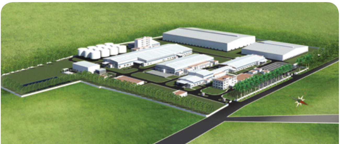
Integrated Food Processing & Logistics Facility, Kapurthala, Punjab (under construction)
