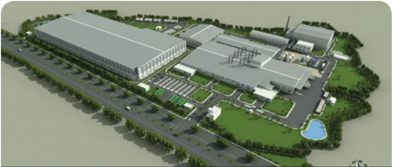
Integrated Food Processing & Logistics Facility, Panchla, West Bengal (near completion)
