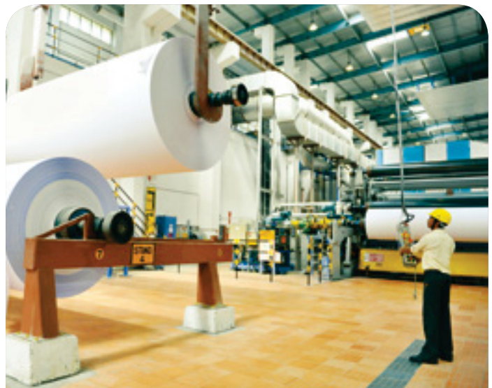
Paperboards Manufacturing Plant, Bhadrachalam, Telangana
