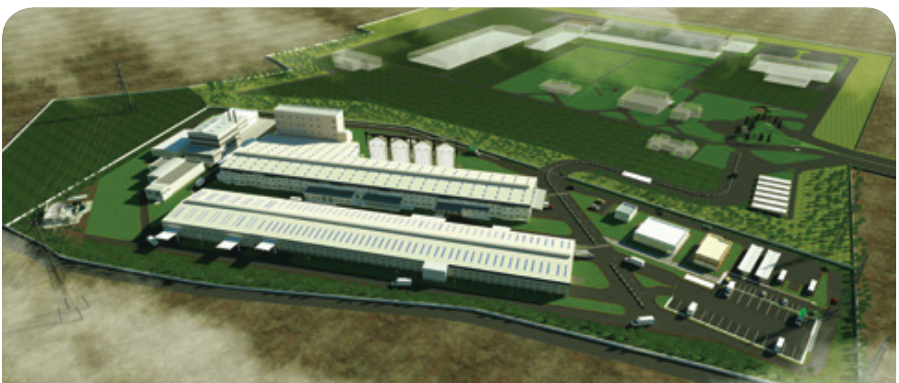
Foods Factory, Mysuru, Karnataka (under construction)
