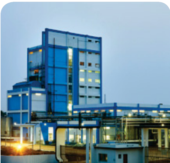
Dairy Plant, Munger, Bihar
